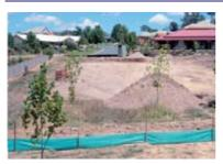
Stockpiles and construction materials are not allowed to be stored on the footpath or within the road reserve without Council permission. Where necessary, stockpile losses can be minimised with the use of covers. All stockpiles and construction materials should be located within sediment controls.
