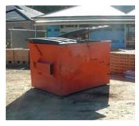
All hard waste must be stored on-site in a way that prevents material loss caused by wind or water. Smaller materials such as litter should be contained in covered bins or litter traps formed on three sides by a geo-textile wind break.
