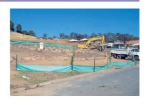
from their support posts during working hours to allow the unloading of materials. For reasons of public safety and sediment controls efficiency, sediment barriers should not be located outside property boundaries. Sediment barriers should not be placed on the road. Sediment barriers placed in front of roadside stormwater inlets are rarely effective and at best usually result in the sediment being washed down the street and into the nearest open gully inlet.
