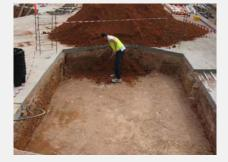
Excavation of one of the permeable tree pit sections
