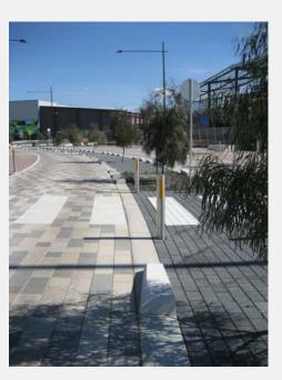
The inverted road profile allows the collection of stormwater in the centre of the road and facilitates the conveyance of larger floods (photo courtesy of Hume City Council)
