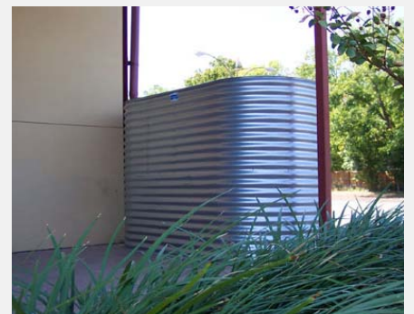
Metal rainwater tank
