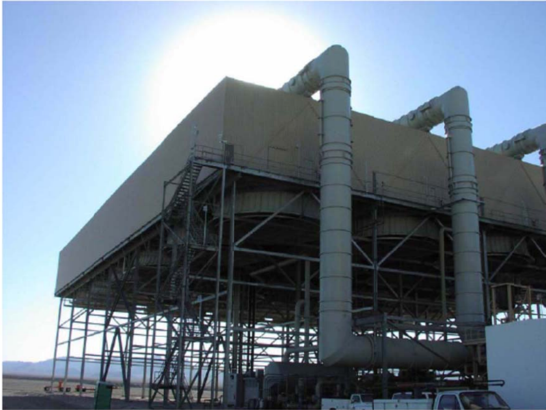
Figure 9 Air-cooled cooling system at El Dorado generating station [2]
