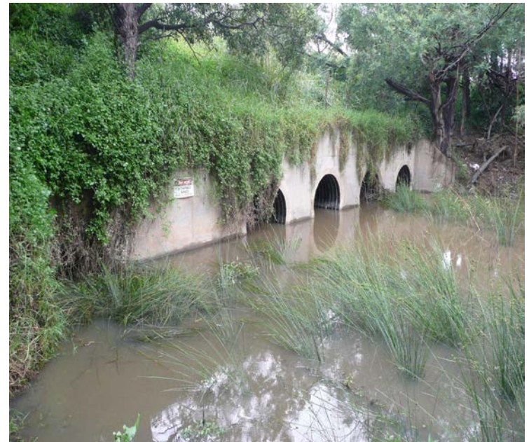
Outlet to Bulleen culverts (27/11/2010)
