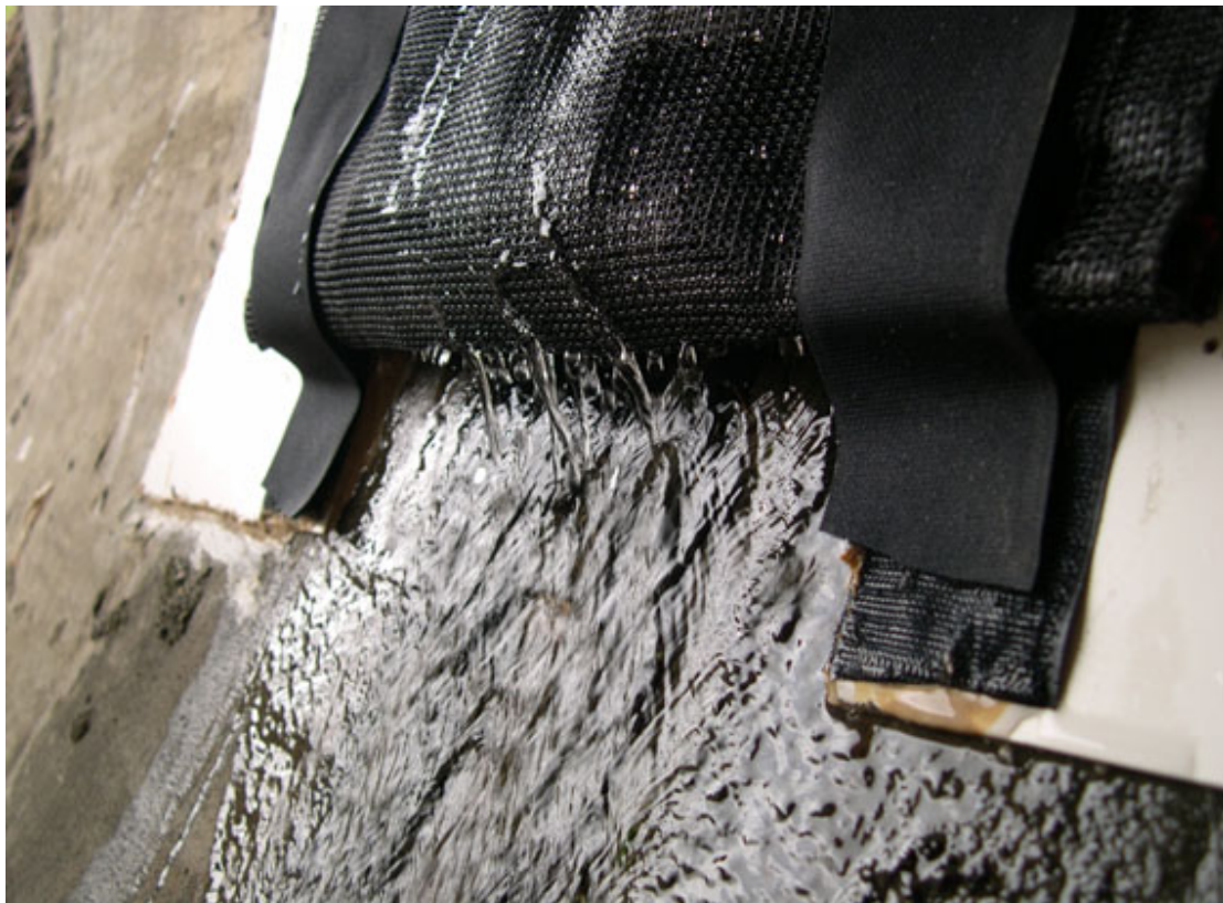
A porous bag containing GAC anchored across a discharging stormwater drain.
