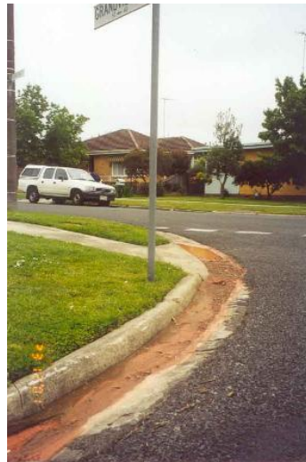
Figure 4. Sediment from brick cutting not being managed
