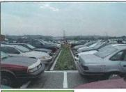
Bioretention System for all our parks. Typically the bioretention system will consist of a 0.3 to 0.5 m wide trench, weappat with a geoscatile father and filled with a prescribed filtration media (sandy loom), planted with obested landscape plants. The filler medium is kept free-thairing with a sketted pipe undertrain which connects in conventional stormwater pipes.
