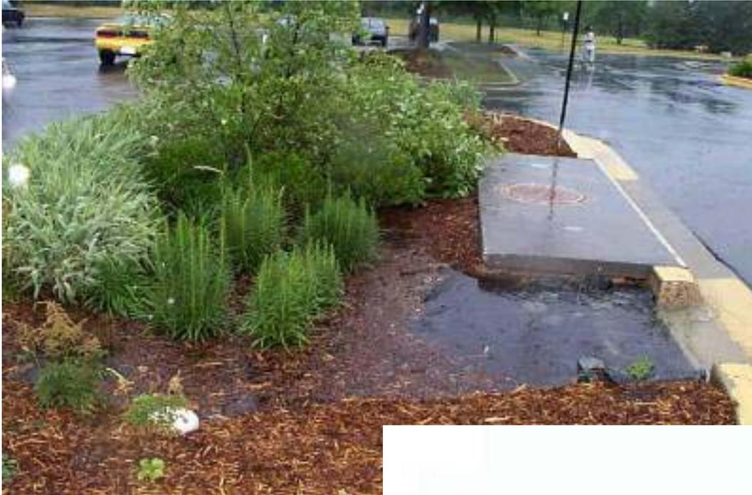
**Bioretention provides stormwater infiltration, retention and treatment**
