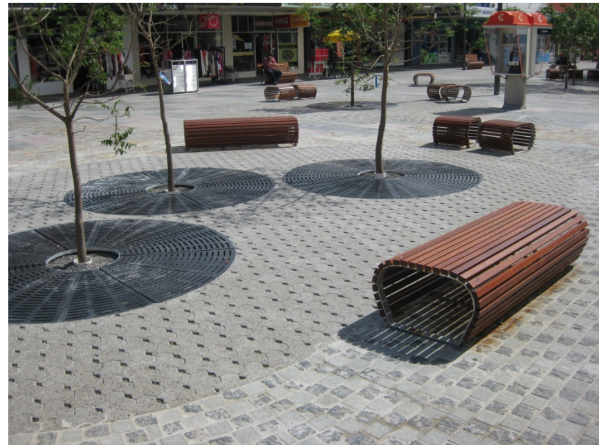
Langtree Mall Tree Pits and permeable paving, Mildura
