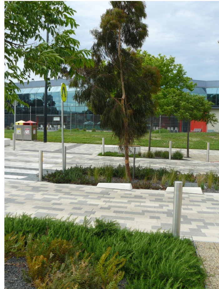
Bio-filtration swales integrated into the streetscape
