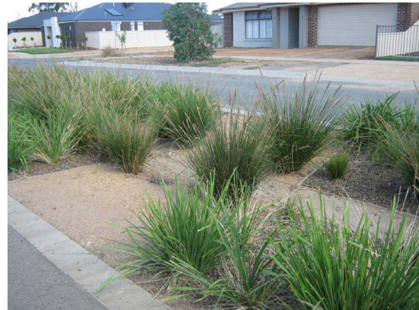
Bio-filtration swales integrated into the streetscape All case study images courtesy of CPG Australia
