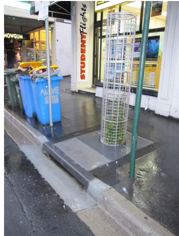
Glenferrie Road Climbing Pit – establishment phase Image courtesy of the City of Boroondara
