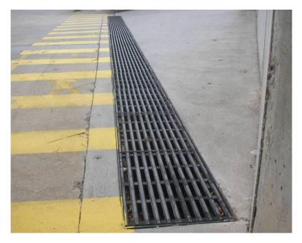
Figure 7. Example of a trench grate
