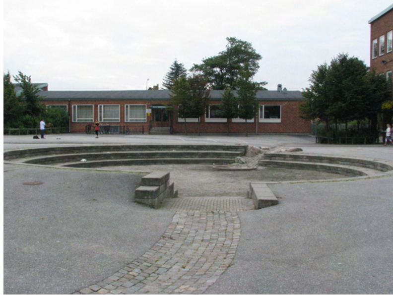
Figure 15: Filtration basin in school grounds, Malmö, Sweden
