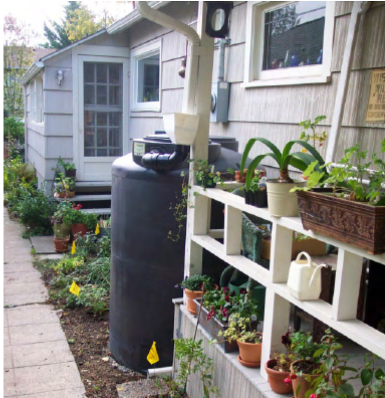
Figure 4: Rainwater tank retro-fitted to dwelling (Mills, 2008)
