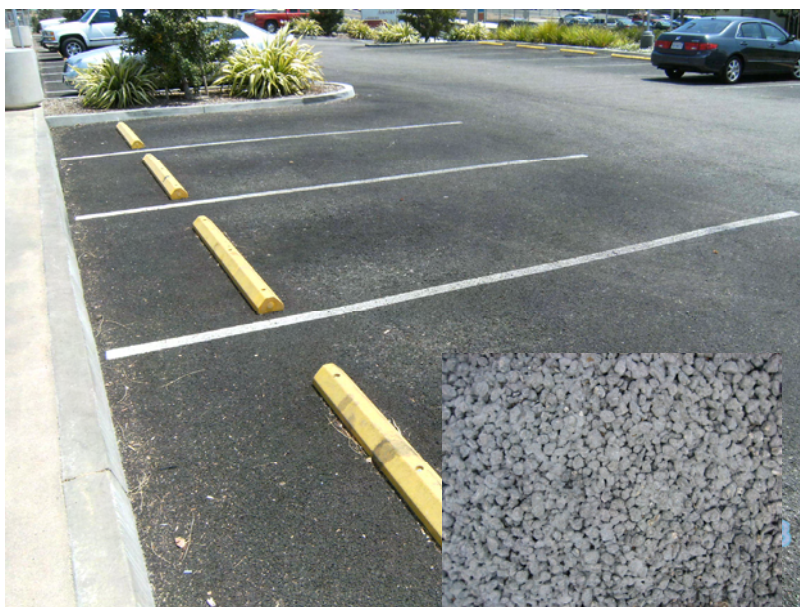
Figure 8: Asphalt porous pavement in car park, Santa Monica, USA;
