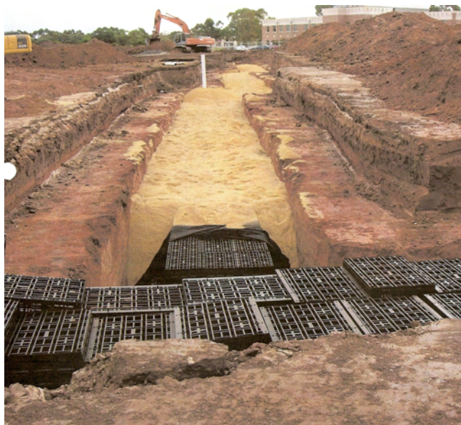
Figure 18: Storage cubes that are used to for storage to any size required (Ausdrain Stormwater Solutions, 2006)
