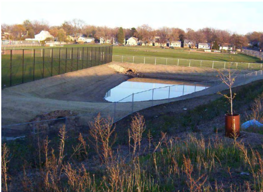
Figure 14: Common stormwater basin (Kelly & Sipalia, 2008)
