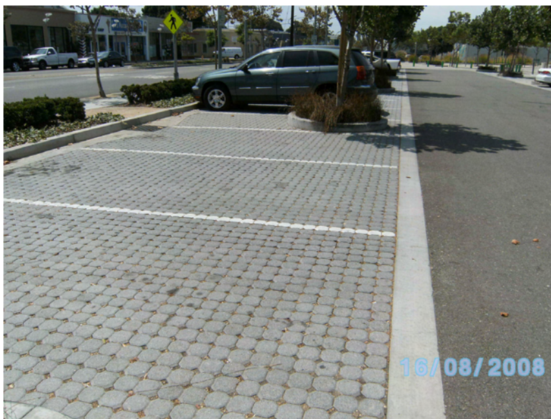
Figure 7: Interlocking porous paving in car park, Santa Monica, USA
