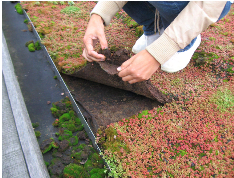
Figure 12: Extensive roof garden, Malmö, Sweden
