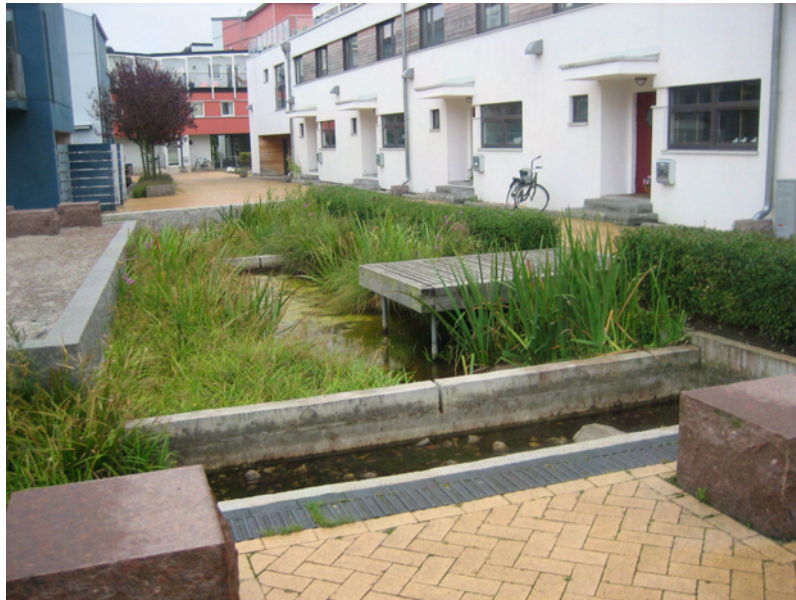
Figure 3: Water Sensitive Urban Design, Malmö, Sweden
