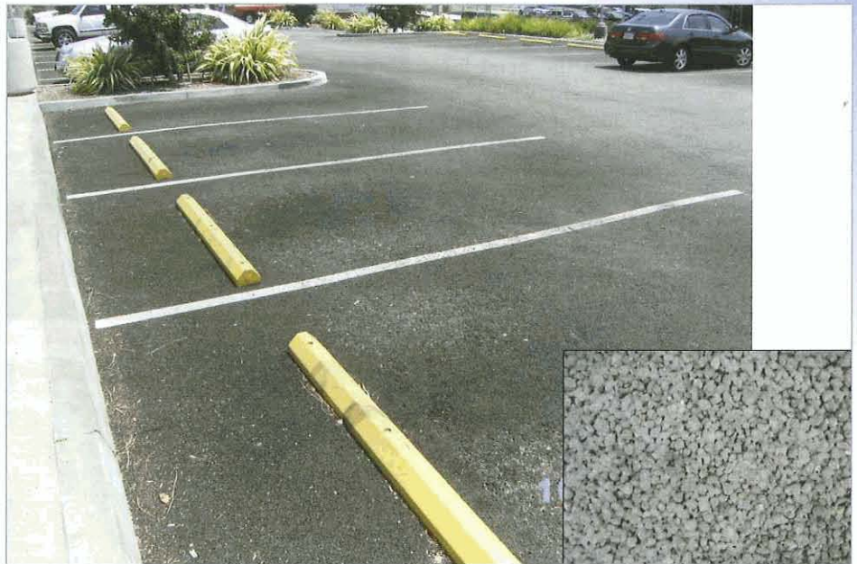
Figure 2. Asphalt porous car park pavement, USA; insert: Porous concrete mix.
