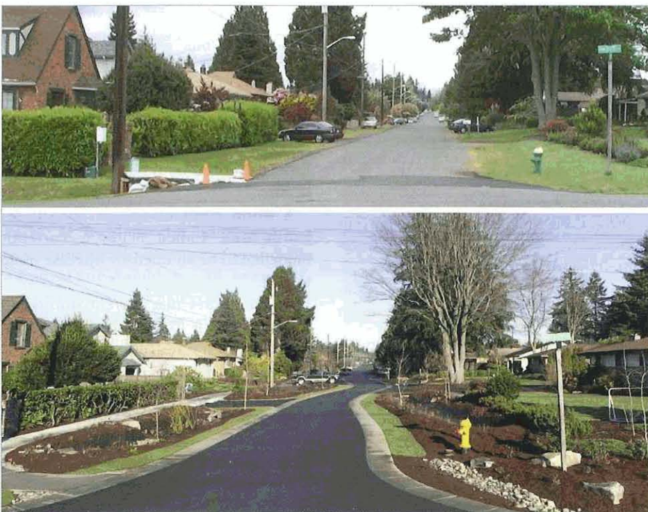
Figure 3. Reconstruction of a roadway, USA
