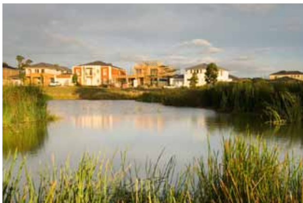
Figure B-7: Pond system with edge vegetation Source: Melbourne Water.
