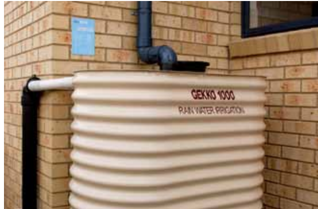
Figure B-8: Rainwater tank Source: Melbourne Water.
