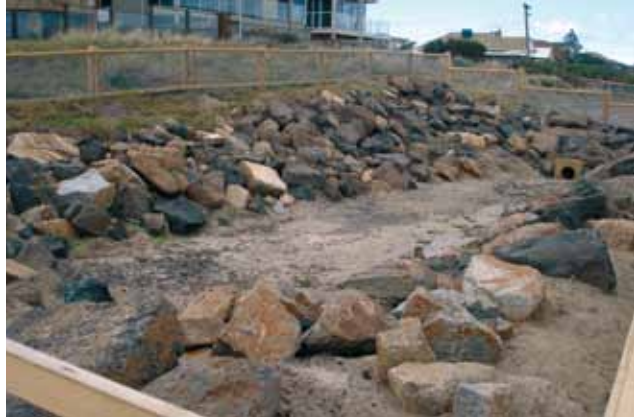
Figure B-4: Sand Filter Source: Melbourne Water.
