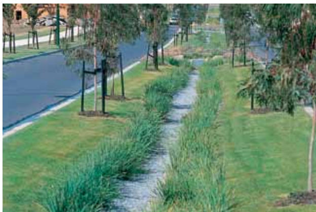
Figure B-3: Vegetated Swale Source: Melbourne Water.
