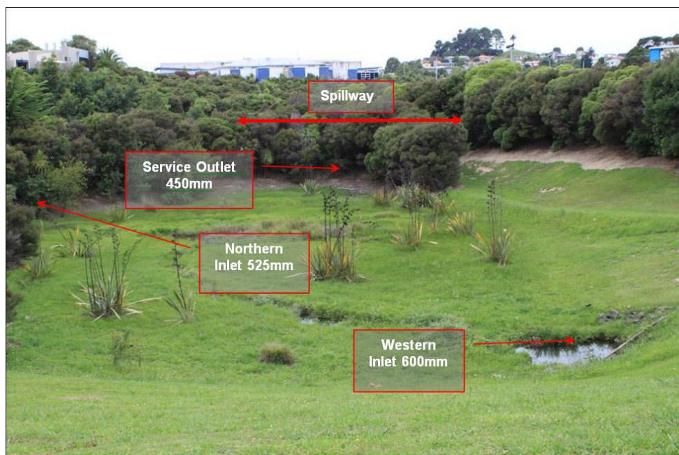
Figure 4: Showing Pre Works Omega Pond (facing East)
