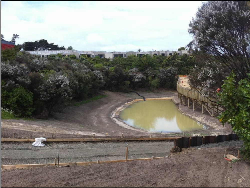
Figure 9: Omega Pond Showing Construction of Deep Water Forebay
