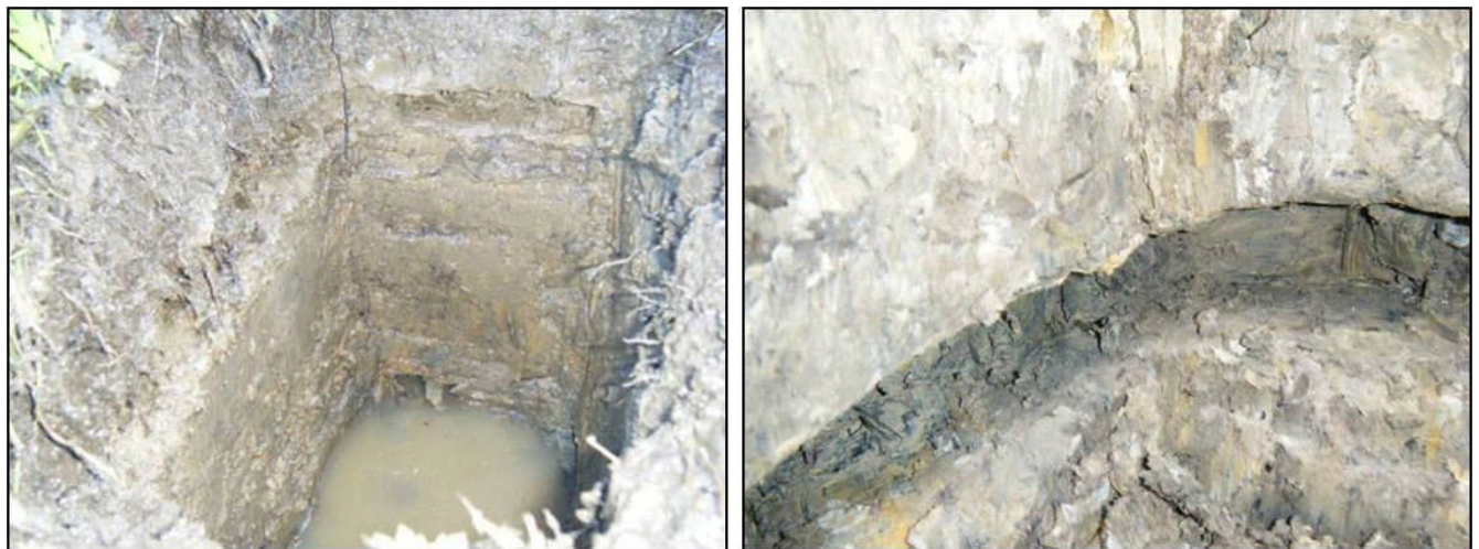
Figure 5: Showing Test Pits Dug into Accumulated Sediment
