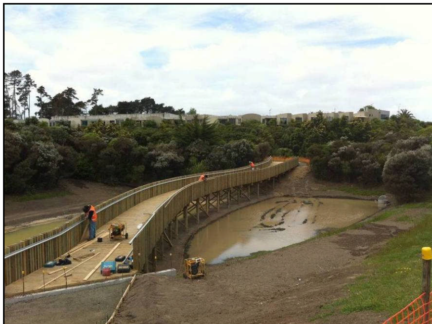
Figure 10: Cycle-way Developed on top of the Separation Bund.
